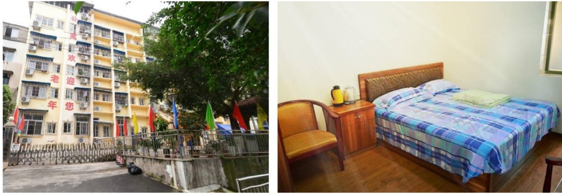
Figure 1: The case study building (left) and a typical room (right)
